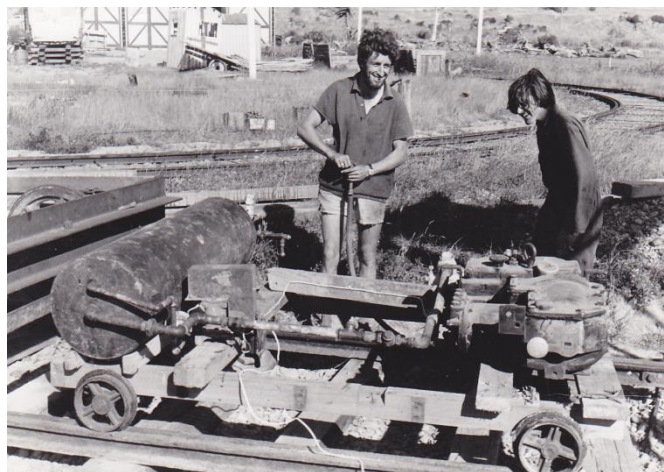
THREE PHOTOS: The Kitson steam tram reprised its former maintenance role with the CTB, helping assemble the new overhead with the help of two special wagons, the homemade tower wagon referred to by Dave Hansen below and the 'Circus' ballast wagon mounted on a Brill Radiax trailer truck, still in use in a modified form 50 years later! Also in use at the time, the trolley-mounted compressor, predecessor to the Society's current work tram 5W, both of which were constructed by Steve Lea, seen here with a very young Greg Harris. Photos: Dave Hinman.
