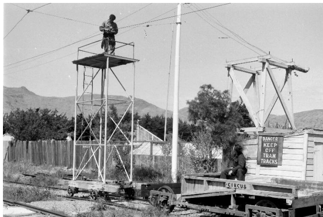
THREE PHOTOS: The Kitson steam tram reprised its former maintenance role with the CTB, helping assemble the new overhead with the help of two special wagons, the homemade tower wagon referred to by Dave Hansen below and the 'Circus' ballast wagon mounted on a Brill Radiax trailer truck, still in use in a modified form 50 years later! Also in use at the time, the trolley-mounted compressor, predecessor to the Society's current work tram 5W, both of which were constructed by Steve Lea, seen here with a very young Greg Harris. Photos: Dave Hinman.
