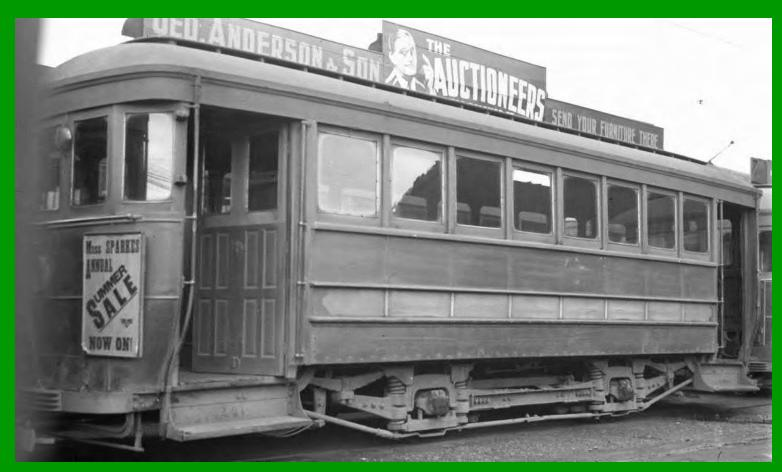
**ABOVE:** 'Standard' trailer 140 stands in the trailer sidings at the Falsgrave Street depot, October 1951. This trailer was one of seventeen (Nos. 126-142) that were equipped with Peckham P21 trucks built by local firm Cooper & Duncan, the others being fitted with Brill 'Radiax E-1' (Nos. 146-149, 201-206). Photo: Graham Stewart.
