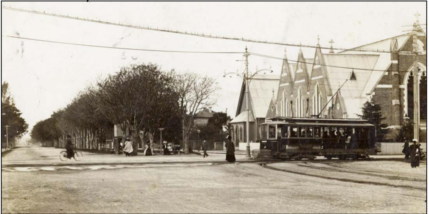
Above: Ken Henderson came upon this interesting photo of a Yank crossing Bealey Avenue en route to Papanui. The photo must have been taken just before the Fendalton line was opened as the rails are in place into Bealey Avenue but there is no overhead.
