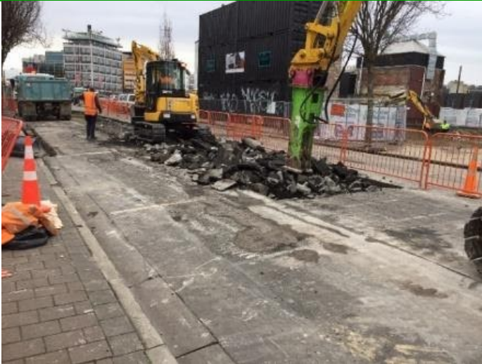
ABOVE: Fulton Hogan work crews expose and remove some of the last remaining sections of ex-CTB tramway rail in High Street along the route of the tramway extension, 15/07/21. Two photos: Dave Hinman.
