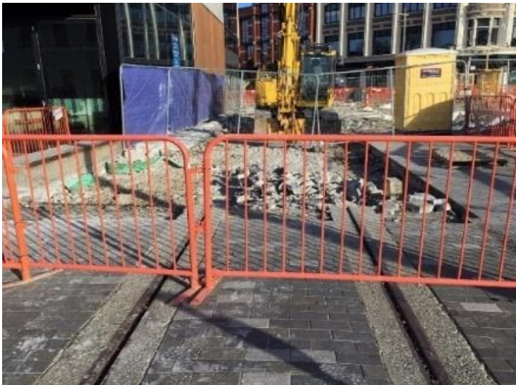
ABOVE: Fulton Hogan work crews expose and remove some of the last remaining sections of ex-CTB tramway rail in High Street along the route of the tramway extension, 15/07/21. Two photos: Dave Hinman.
