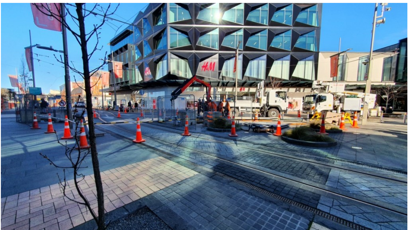
BELOW: Being done at the same time as the extension works and the anti-terror bollards in Oxford Terrace, CTL have installed two new traction poles at the High Street-Cashel Street intersection. This was the scene on July 28 as contractors removed the existing paving to make way for the poles. Photo: Stephen Taylor.
