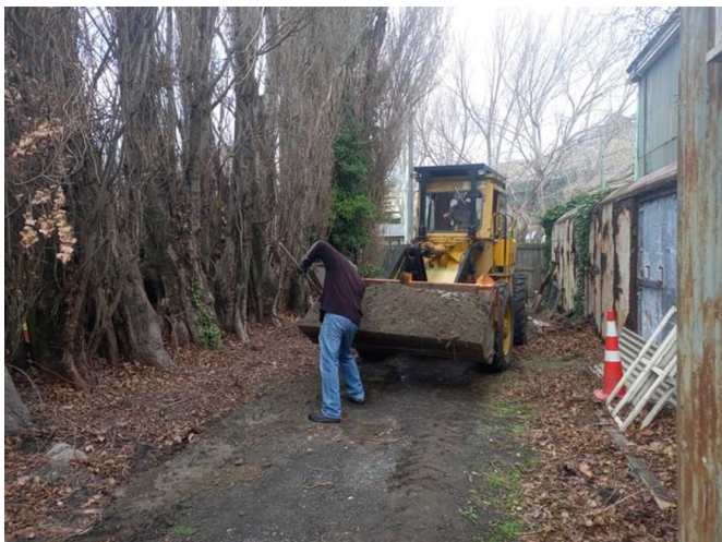
ABOVE: Philip and Mark spreading more pit run along the east side of the Trolleybus Shed with the CRS loader.
