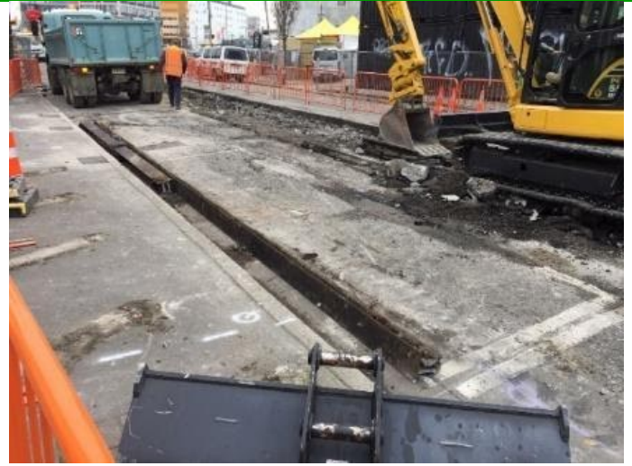
ABOVE: Fulton Hogan work crews expose and remove some of the last remaining sections of ex-CTB tramway rail in High Street along the route of the tramway extension, 15/07/21. Two photos: Dave Hinman.
