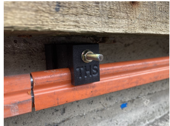
Top photo: Callum installing the new hanger system (Photo Ken Henderson)
